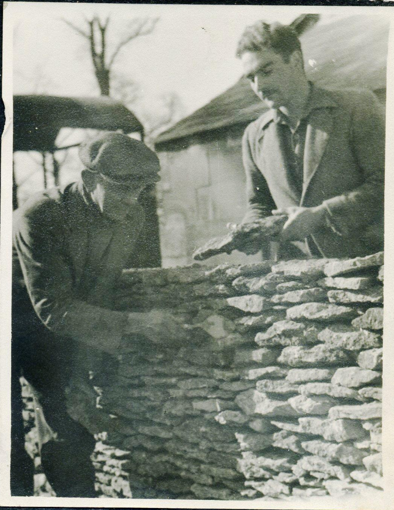
Henry Cole who worked for Lord Glanely and Major Holt, dry stone walling at Home Farm, 1950. He was responsible for building the wall on the road side enclosing Wall Field, Biddestone Lane.
