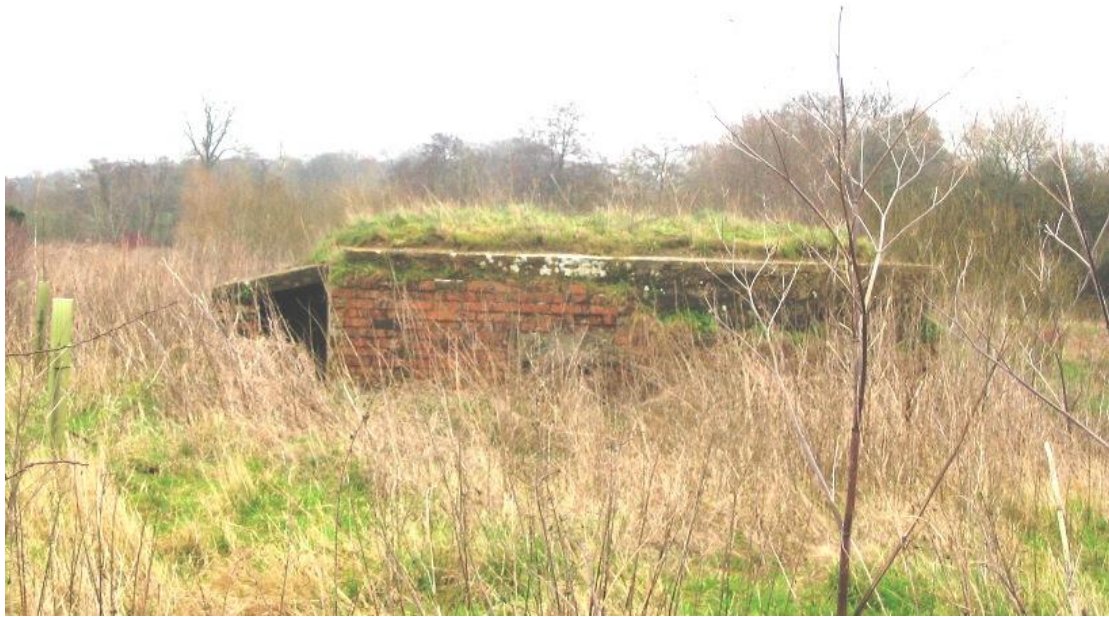
1.1 View from the south west, R. Avon to the right
