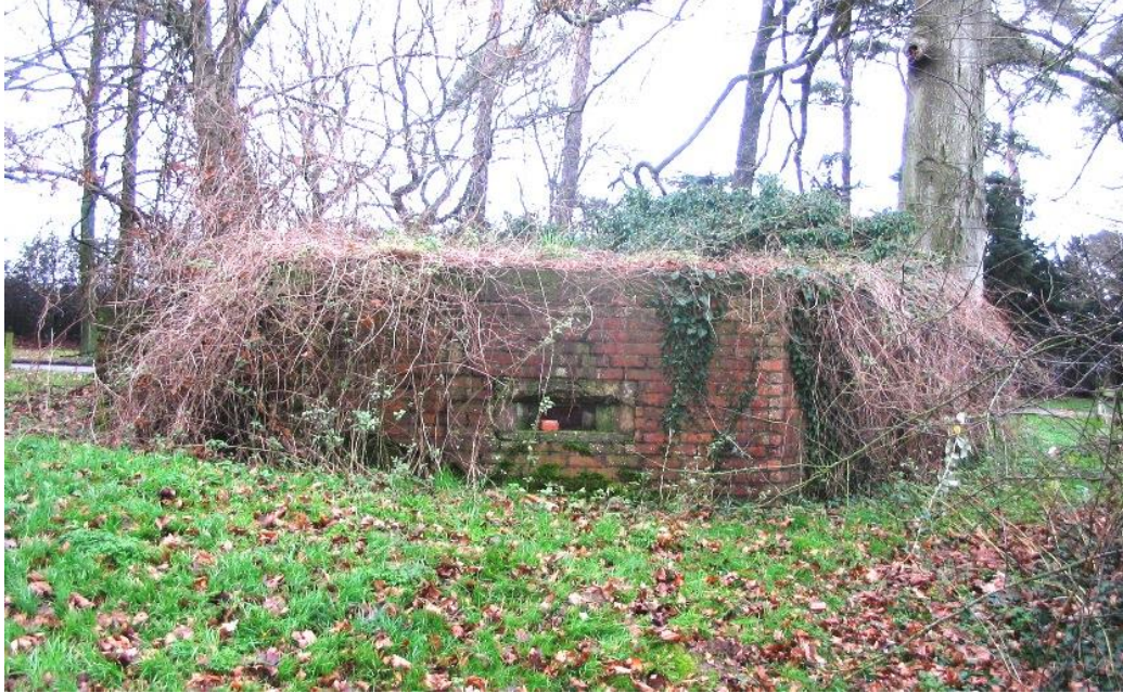
5.1 View from the south east
