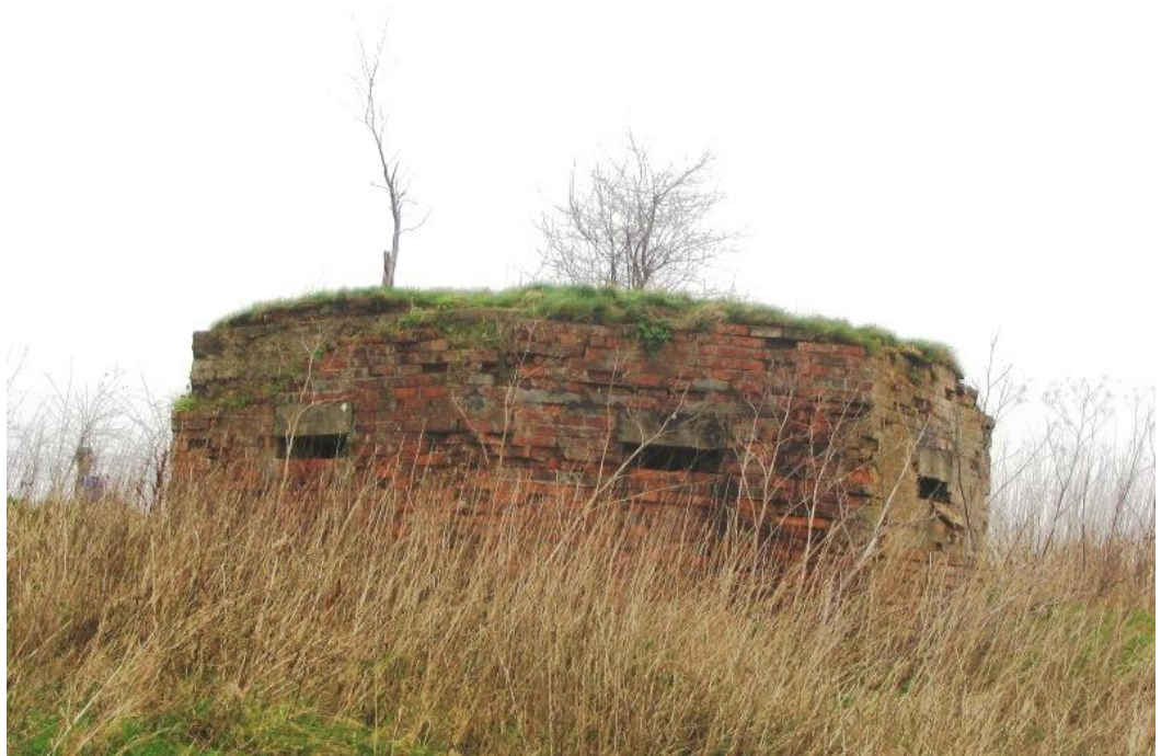
2.2 View from the bank of the River Avon looking north east
