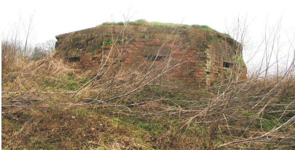
1.2 View from the bank of the River Avon looking north east
