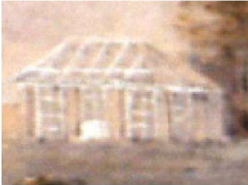
Fig. 23 Summer house 1844 [detail from Fig 20] **
