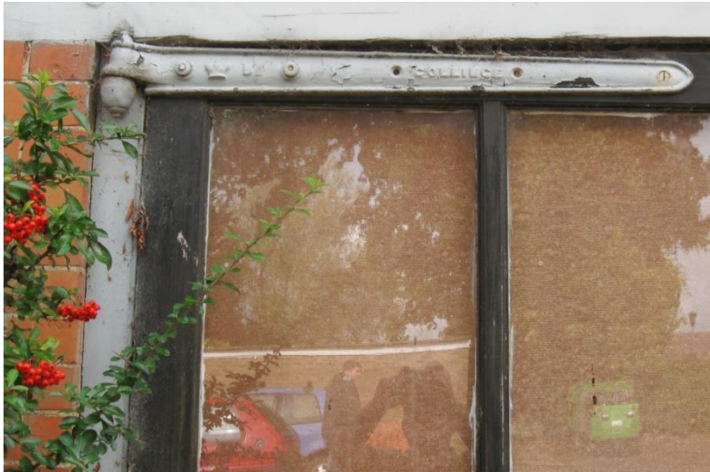
Fig. 55 a) Collinge hinge in place on the doors a) before renovation
