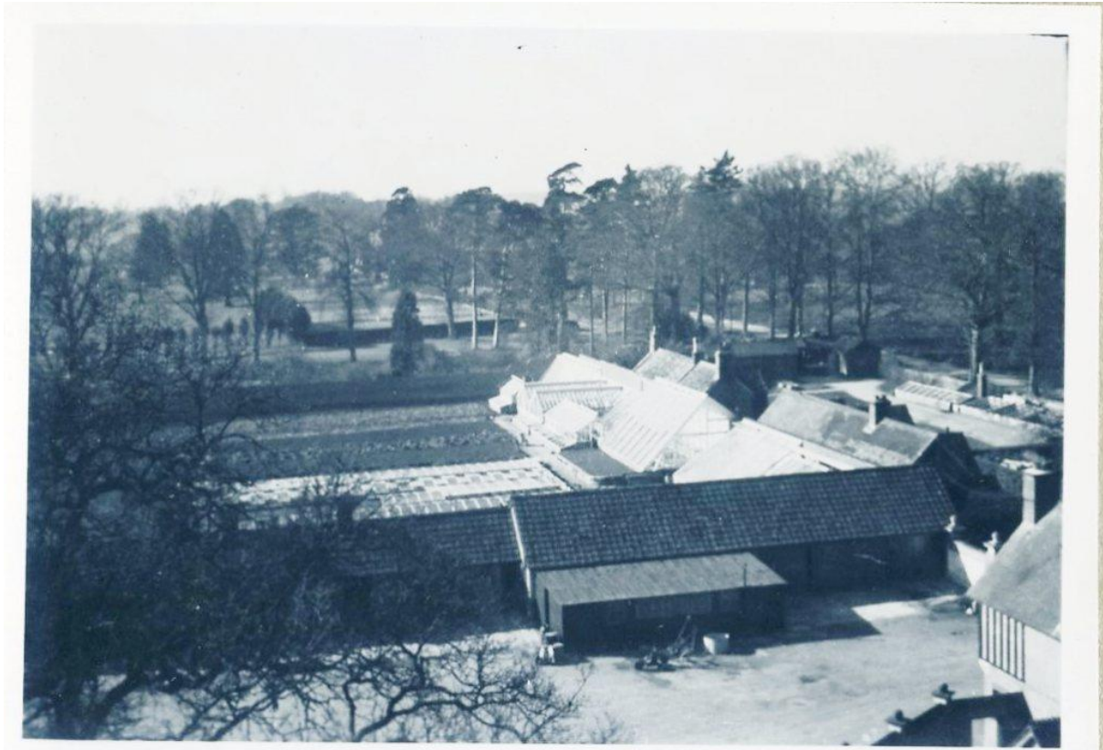
Fig 3 Photograph taken from the top of the water tower looking north west 10 towards Lackham House
